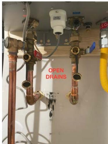
To get the unit back up and running reverse process above. Before plugging in unit and turning it back on you MUST turn on a faucet or fixture to hot and let water run while starting unit to fill heat exchanger so it doesn't burn up.
